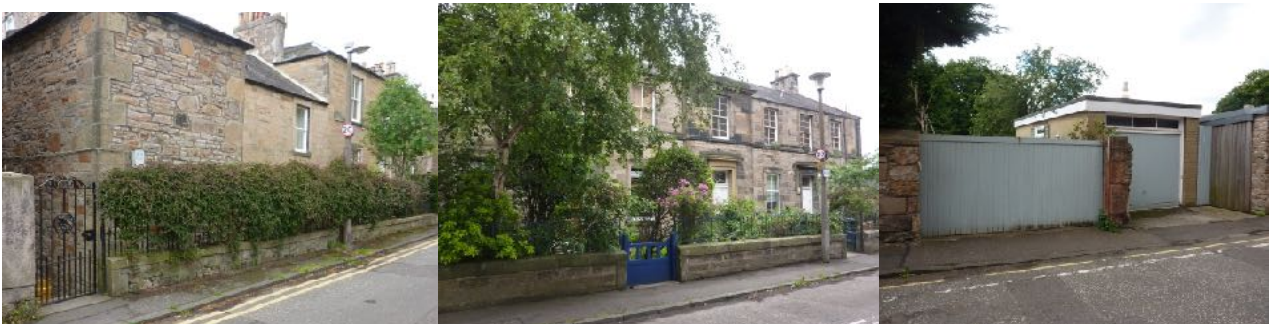
Rear elevation (no.13) versus front elevation (no.8-10), and existing less welcoming parking strategies on Jordan Lane
