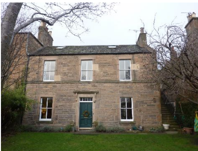
Front elevation of 13 Jordan Lane, facing south
