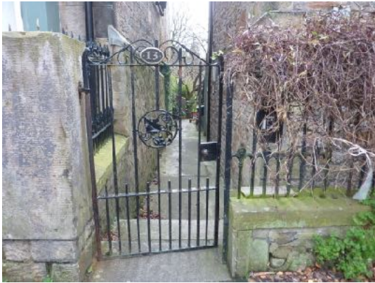
Existing narrow gate and sudden drop in level at entrance to 13 Jordan Lane
